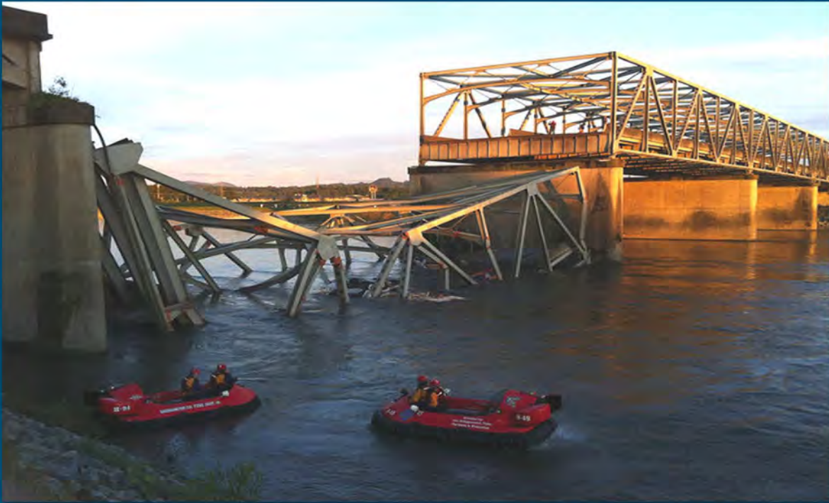
SEARCH AND RESCUE Washington Bridge, Snohomish County FD
